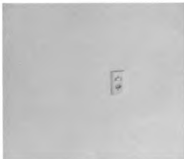
Figura 12 – Interruptor com tomada
